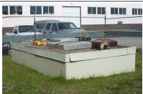
Photo 6: Well No. 11 Pump House
