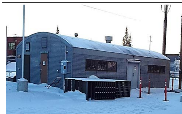
Photo 3: Building J-5 (also known as Building 607)
