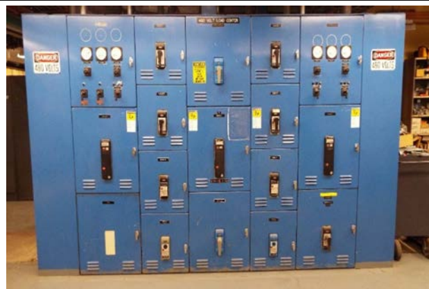
Photo 1: Electrical switchgear in Building 606 North
