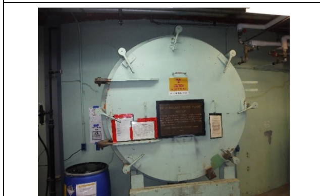
Photo 5: VC access hatch inside Building 606 North
