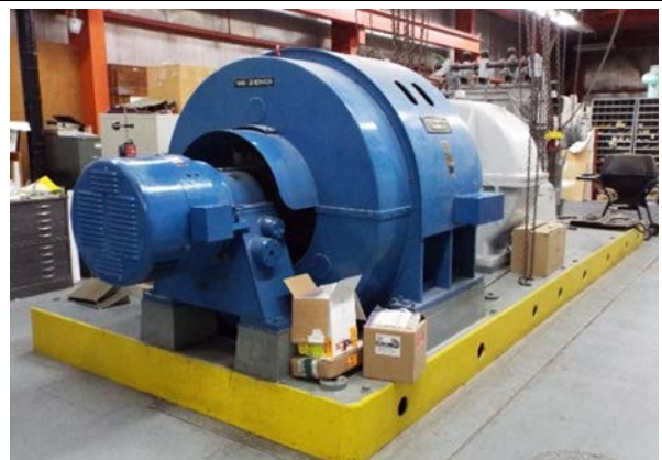
Photo 2: Electrical generator (foreground, blue) and turbine (behind generator at right) associated with the original operation of SM-1A in Building 606 North
